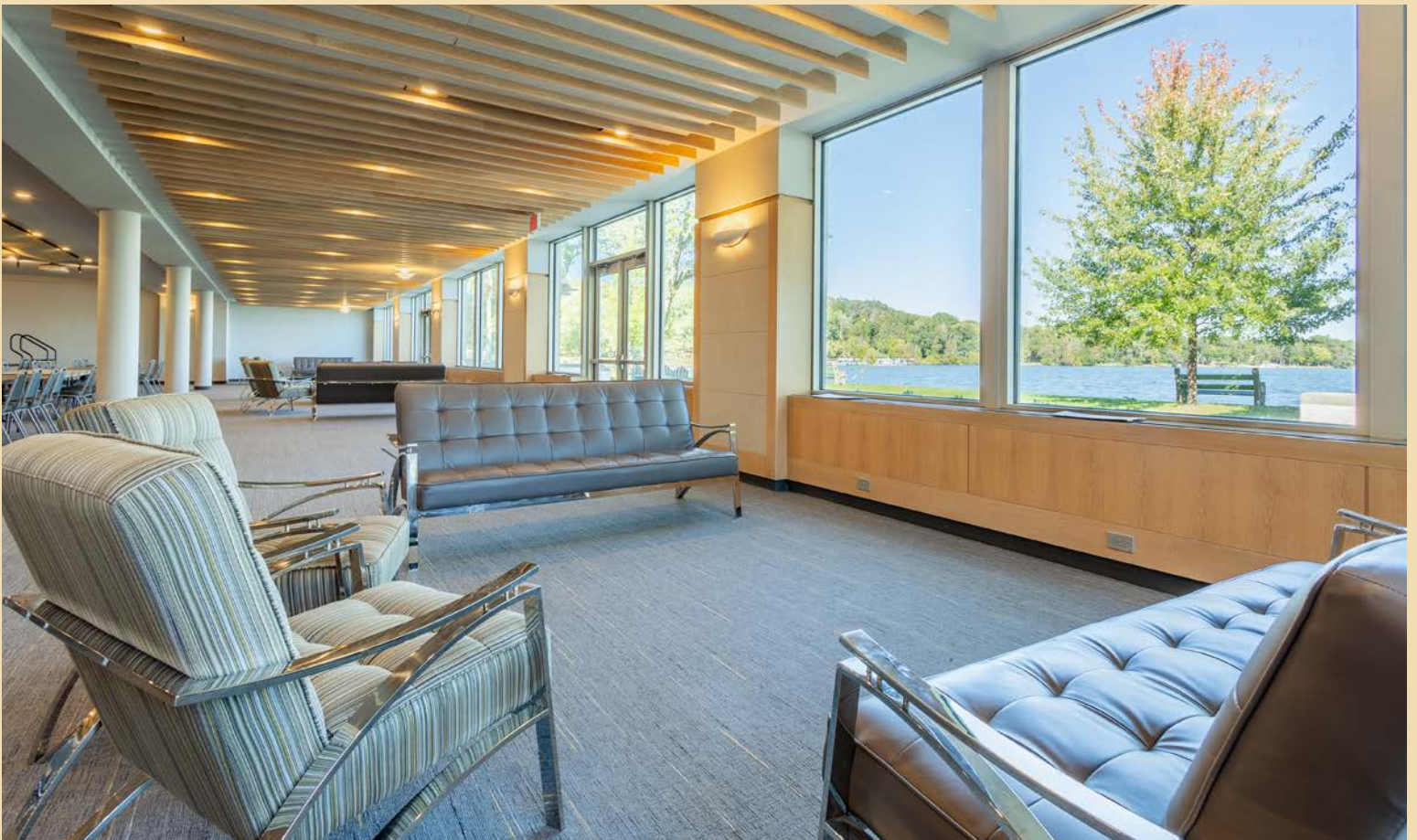
Large new windows and doors offering unobstructed views of the lake were installed in Staughton Hall.
